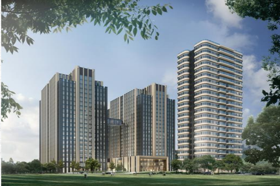
New Construction of Formosa Plastics Building Urban Renewal
